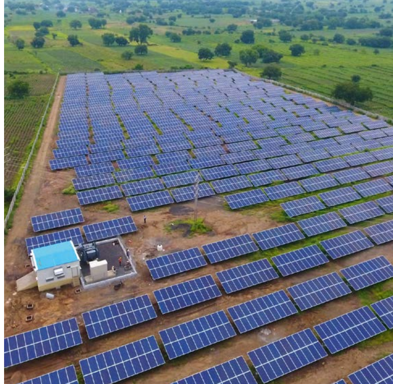
Aerial view of Mirkala Solar site.
